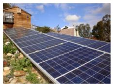
Multicrystalline 2.8 kW, the Phase 2 is ground-mounted.
