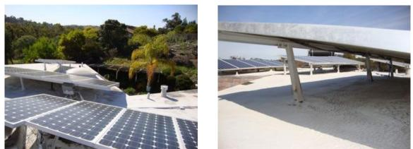
After the <u>rooftop PV</u> & solar hot water in 2003, we installed foam on our flat rooftop. This white foam reflects sun in Hot Summers helping cool our building, and is an insulator in Winters like snow helping hold in warmth. This is reducing energy use year-round. Moreover it is keeping rain from seeping through the flat roof, a side benefit.
